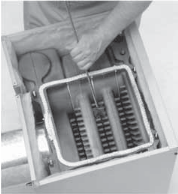
Figure 22 Thoroughly clean flueways between all pins at all angles. Start on top of boiler, finish from the bottom.
