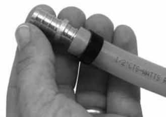
CrimpRing and fitting installed on RadiantPEX tubing.
