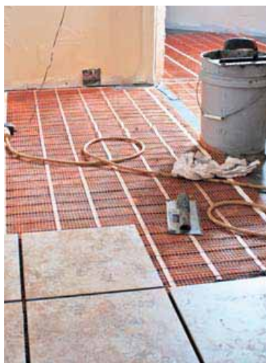
Trowel thin-set and lay tile.
