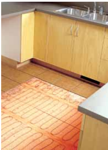
Trowel thin-set and lay tile.
