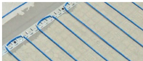
WarmWire installed using CableStrap
