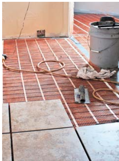
Trowel thin-set and lay tile.
