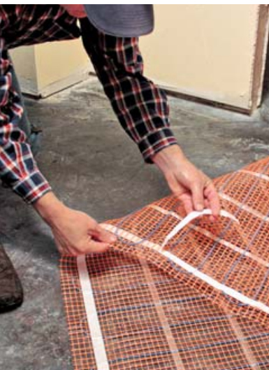
Roll out mat and secure to the floor.
