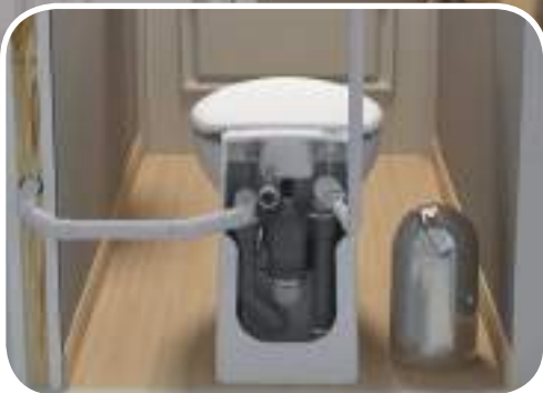
View of installation behind the wall
