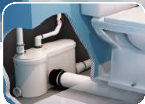
View of installation behind the wall
