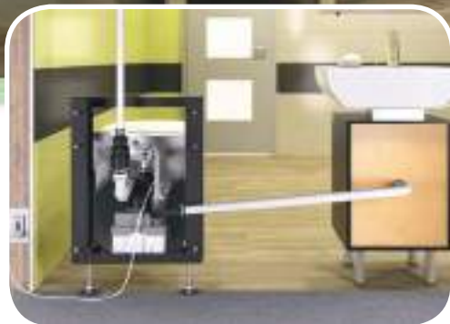
View of installation behind the wall
