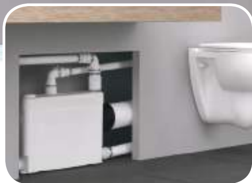
View of installation behind the wall
