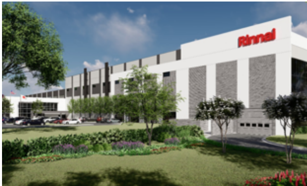
Rinnai Manufacturing Expansion GRIFFIN, GA | OPENING 2021
