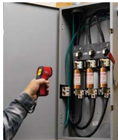
Check fuse or circuit breaker overheating, which could be caused by overloaded circuits.
