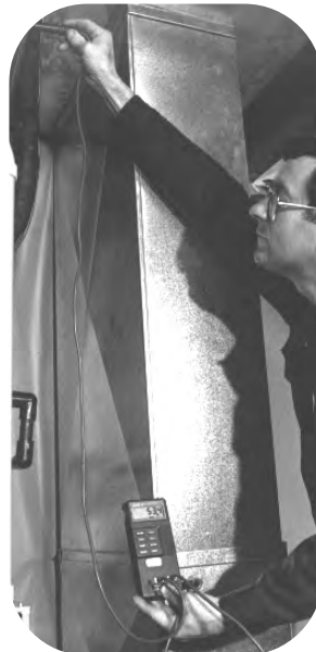
FIGURE 41 TEMPERATURE RISE MEASUREMENT
