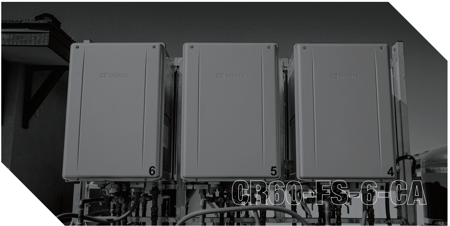
Floor Standing Rack (CDV Units) 6 Water Heaters
