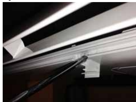
Figure 66: Remove (and Reattachment) Bottom Panel
