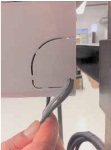
Figure 67: Indoor Unit Knockout (Communication Wires)
