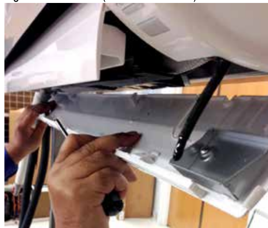
Figure 66: Remove (and Reattachment) Bottom Panel
