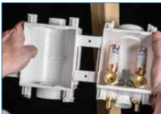
Slide integrated mounting flanges into opposing box
