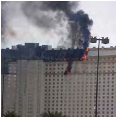
Damage from this hotel fire was contained to the upper floors, but water damage destroyed walls, ceilings, floors, furniture, rugs, artwork, restaurants and stores all the way down to the lower floors.
