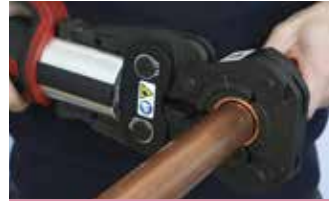
3. Complete the joint with the press tool
