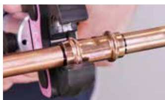
1. Align jaws squarely on the fitting
