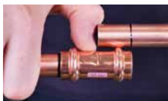
7B. Check the depth mark
