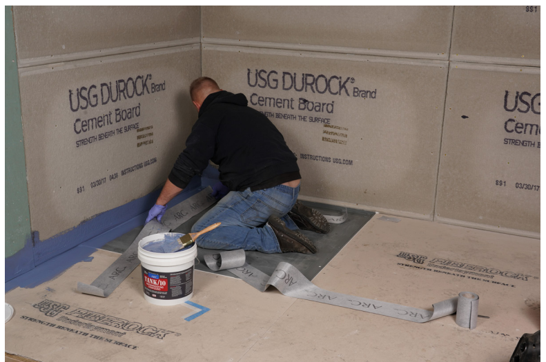
Embedding joint reinforcement tape over floor-to-wall joints.
