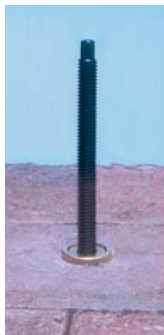
Step 2: Turn stud in anchor.
