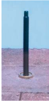
Step 2: Turn stud in anchor.
