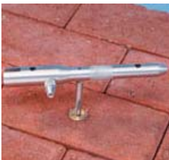
Step 1: Thread anchor with tap.
